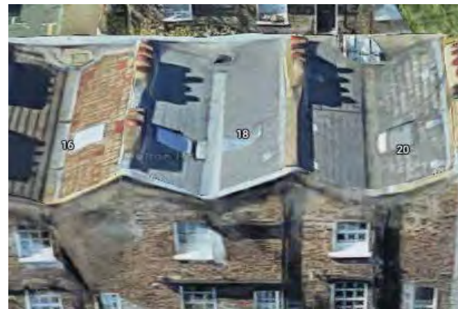
Inverted Pitch roof known as London or Butterfly roof. With V Parapet rear.
