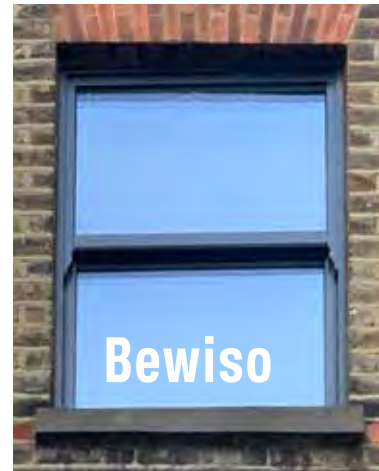
Exterior - Simulated Hung sash Bewiso Victoria - cert. 0.8w/m 2 K
