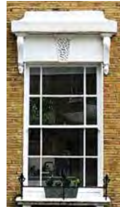
LB of Islington has allowed replacement of the window above in a non listed building with a Slim-Profile double glazed window. (14 Dagmar Terrace granted approval in 23 June 2021).
