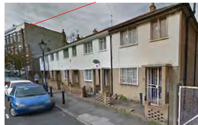
2, 3, 4, 5, 6 Dagmar Terrace /rear garages Lost heritage 4 storey terrace infill with out of scale 2 storey modern terrace damaging the Conservation Area. Poor windows and details suitable for external insulation, new windows, and additional storeys.
