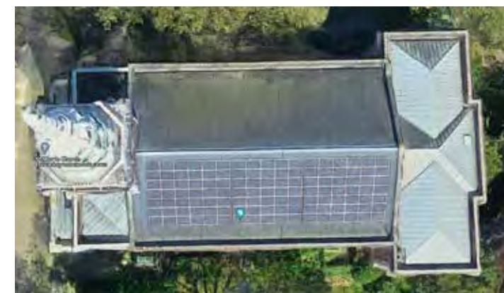
119 panels on St Mary's Church Upper Street
