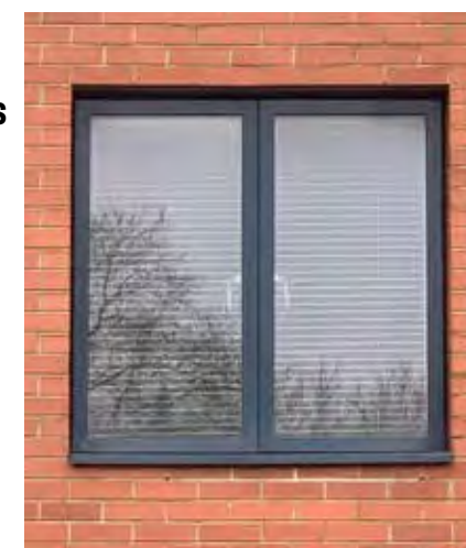
Building nearby outside CA 13
