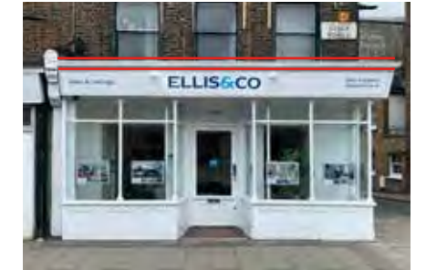
70 Essex Rd, Cornice missing
