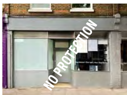
67 Cross St, Fascia Oversize Windows and door rebuild
