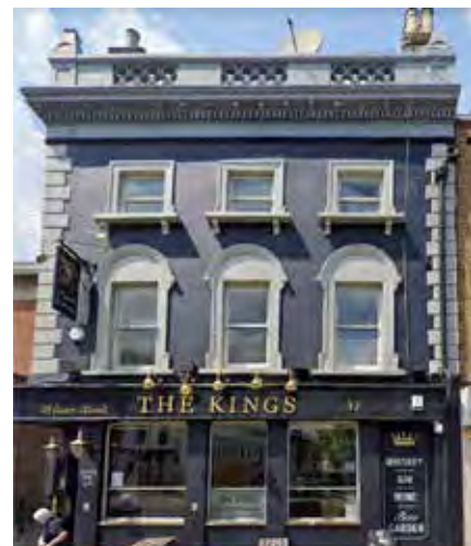
59 Essex Road, suit triple glazed fixed & 1 over 1 sash
