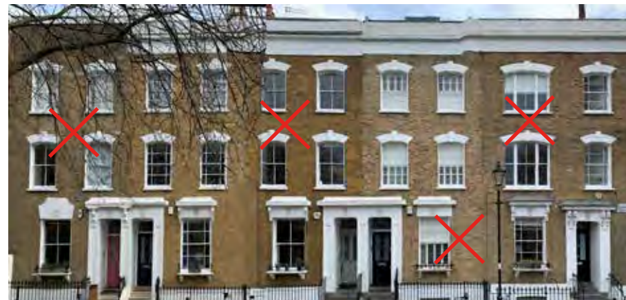
23, 21, 20, and 19 Dagmar Terrace non period windows suit replacement
