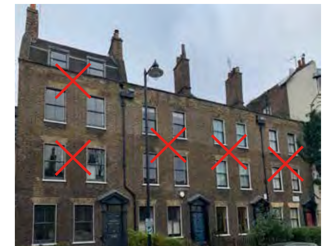
53, 55, 57, 59 Cross Street, 6 over 6 replaced with 2 over 2 Victorian with modern replica wavy glass
