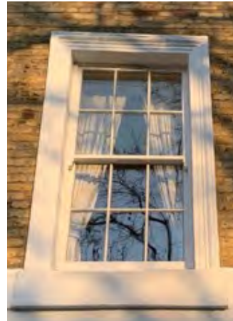
Timber double glazed no secondary reflection within a nearby Islington Conservation Area.
