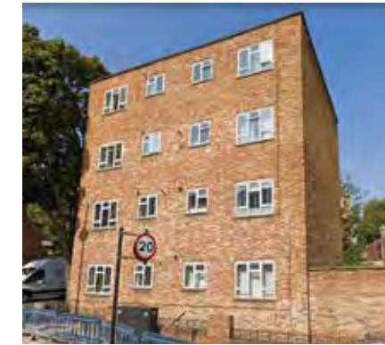
9-16 Fircroft House, Halton Road Poor finishes, PVC windows, and out of scale, suitable for external insulation, new windows, and balcony/ facade extension.
