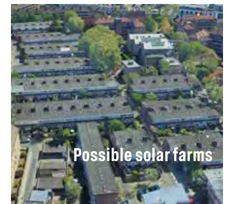
Multiple flat roofs potential Solar farm on council estate
