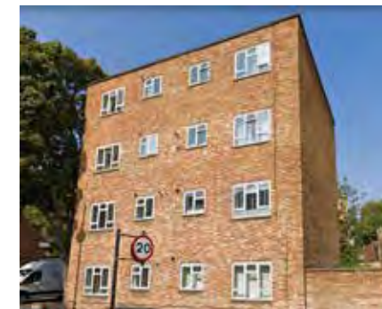
9-16 Fircroft House, Halton Road Poor finishes, PVC windows, and out of scale, suitable for external insulation, new windows, and balcony/ facade extension.
