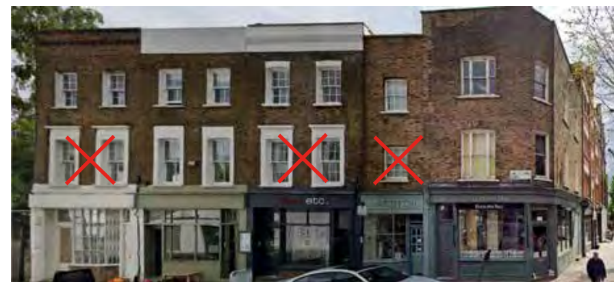
fake Georgian 8, 6, 4, 2 Shillingford Street, 38 Cross Street. Victorian windows have been fake georgianised. All replaced with 1 over 1 triple glazed.
