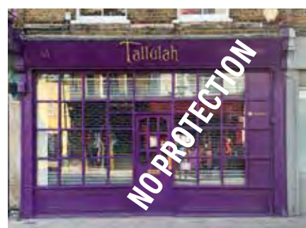
65 Cross St, Fascia Oversize, Windows and door rebuild
