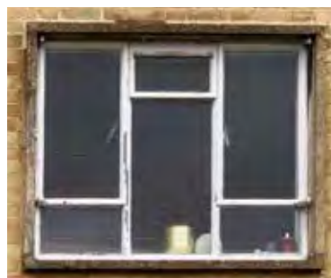
Nearby across Essex Road
