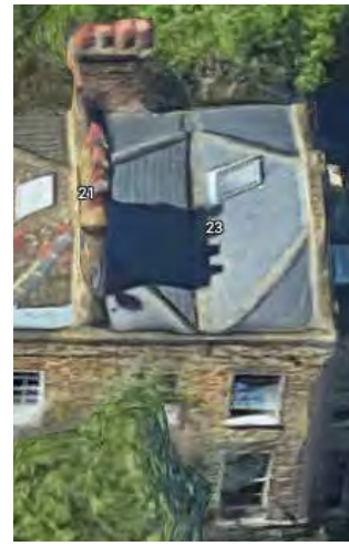
Inverted Pitch- Hip roof. Low front and rear parapets. Roof visible.
