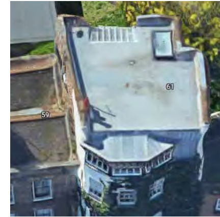
Modern Membrane Flat roof, new floor added to a Listed Building. 61 Cross St
