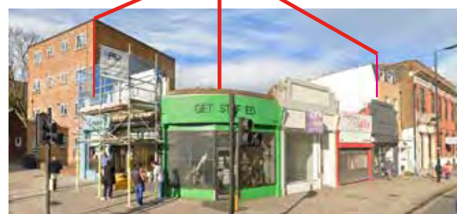
6 shop parade Cross & Essex. Shop fascia and windows damaged, Positive heritage fascia to retain.
