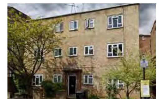
Negative building across Halton street 157
