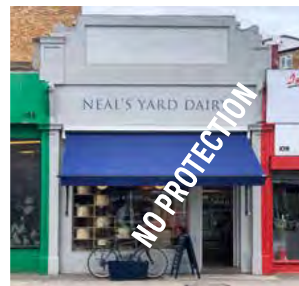
107 Essex Rd, a Unique Parade Pilasters & Brackets should be painted single colour, not split.
