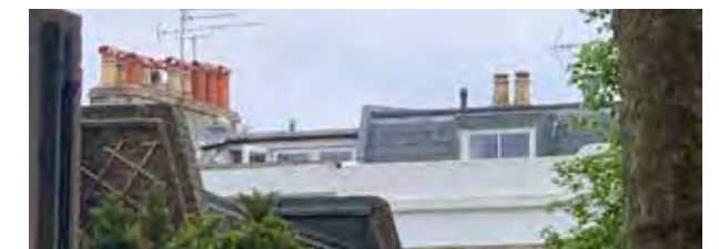
21 & 20 -long view show differing roof heights
