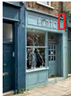
2 Shillingford Rd, Cornice and Brackets missing
