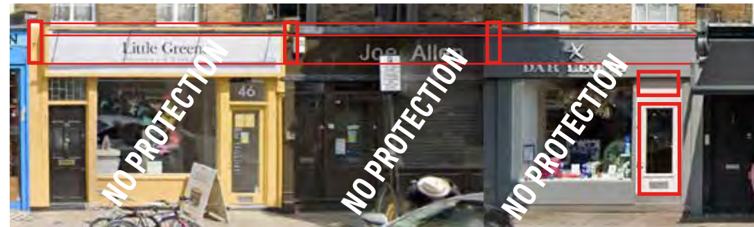
2 Shillingford Rd, Cornice and Brackets missing
