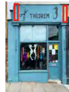
4 & 2 Cross Street, Brackets missing
