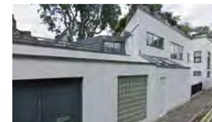
7, 9, 11 Shillingford Street Houses "Developer Modern" suitable for external insulation.
