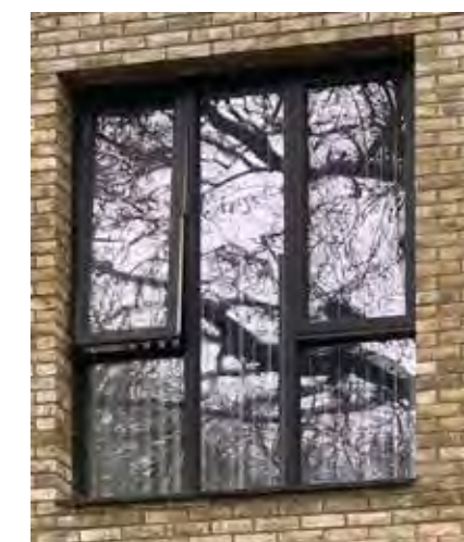
Building nearby outside CA13
