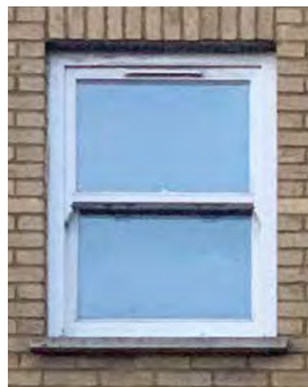
Essex Road, - New build trickle vent slot in top sash
