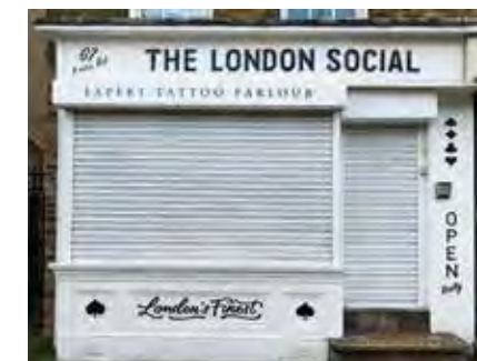
67 Essex Road, roller shutter sign obstructs cornice fascia
