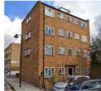
1-8 Fircroft House, Halton Rd Poor finishes, PVC windows, and out of scale, suitable for external insulation, new windows, and balcony/ facade extension.
