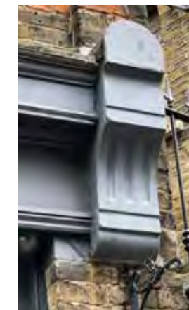
71 Cross Street, CORRECT CORNICE alignment Stepped Fascia
