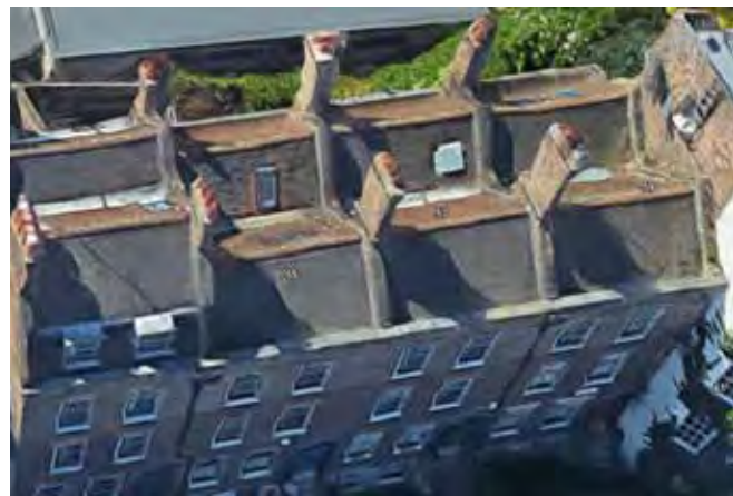
Double Ridge pantiled roof. Ridge parallel to facade
