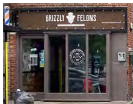
65 Essex Road, solid panel in window area, low stall riser
