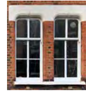
36/34 Cross Street windows
