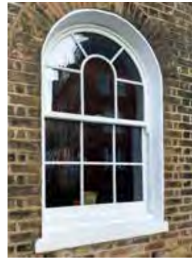
Correct timber slim-profile double glazed slim -profile, Halton Road
