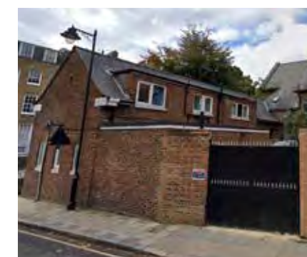
14 Cross Street Low cottage out of scale with terraces suitable for creative extensions.
