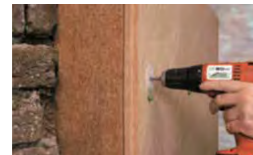
Woodfibre External Wall Insulation i Mineral wool External Wall Insulation install.
