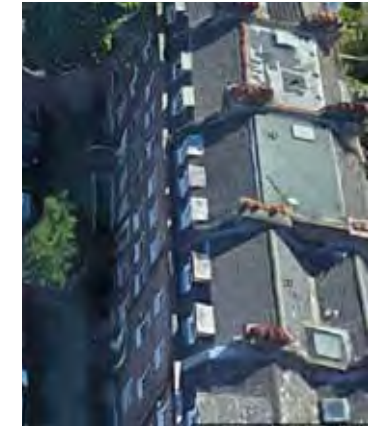
Modern Flat Roof Listed Double Pitch roof infills. Cross Street
