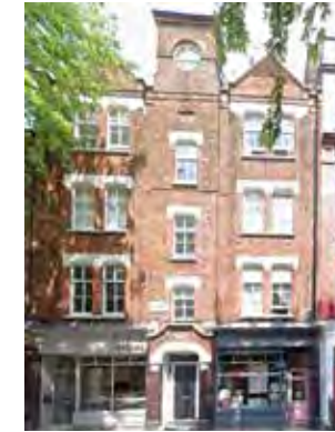
36/34 Cross Street heavy original sash suitable for evacuated double glass panes in the original sash.
