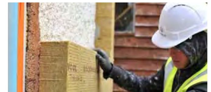
Woodfibre External Wall Insulation i Mineral wool External Wall Insulation install.
