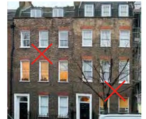
23-29 Cross Street, loss of door pediments on 23,27, & 29 Cross Street
