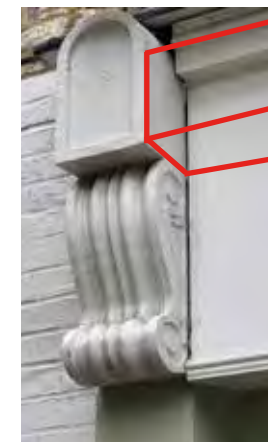
47 Cross Street, Fascia too large, Cornice not aligned with Bracket, bad detail top gaps.
