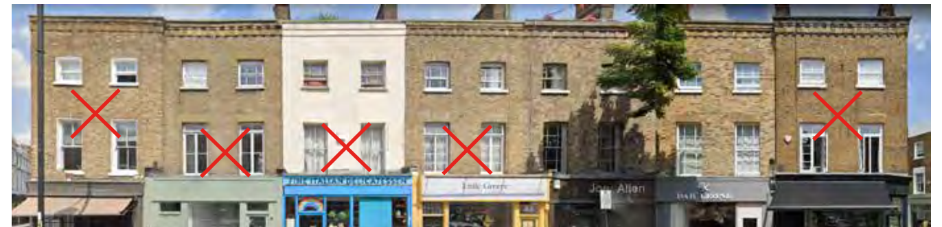
52, 50, 48, 46, 44, 42, 40 Cross Street, Mismatched new windows replace all with double glazed 44 and 42 are correct decorative Victorian type
