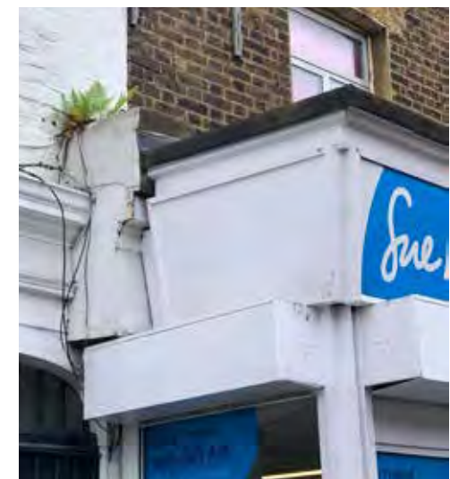
72 Essex Road, shop extension built tight on centre of party wall (or even over the line) not to inside as normal with shops. Roller shutter box extends in front of neighbours window!!
