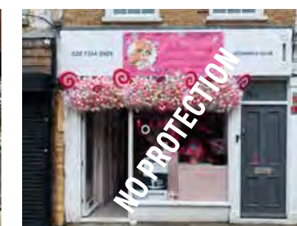
76 Essex Road, sign obstructs cornice and fascia
