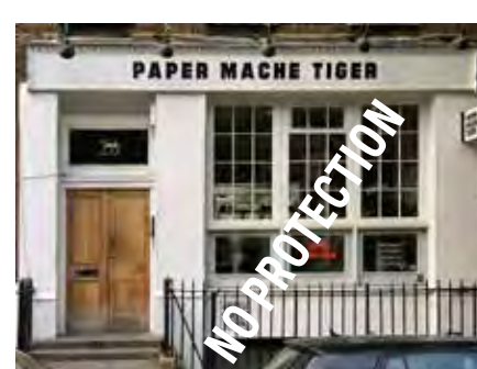
26 Cross St, Roller Shutter, windows damaged
