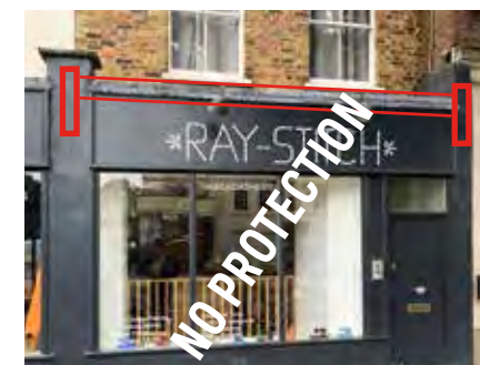
68 & 66 Essex Road, Cornice and Brackets missing
