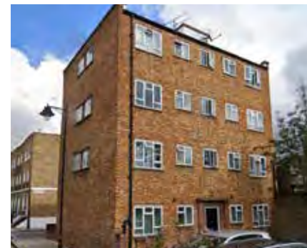
1-8 Fircroft House, Halton Rd Poor finishes, PVC windows, and out of scale, suitable for external insulation, new windows, and balcony/ facade extension.
