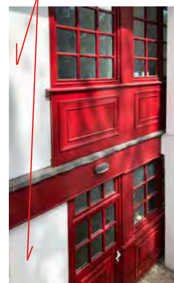
30 Cross St, Recessed Basement window wall. Heritage correct. Double glazed units in old mullions.
