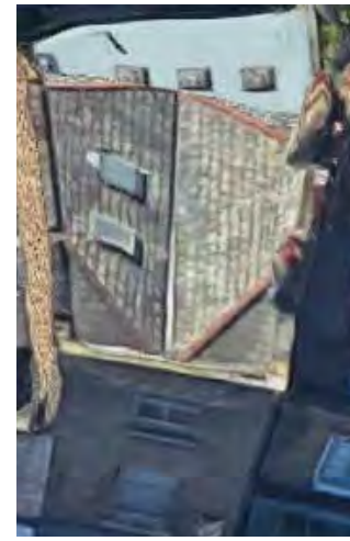
Inverted Pitch- Hip roof. Low front and rear parapets. Roof visible.
