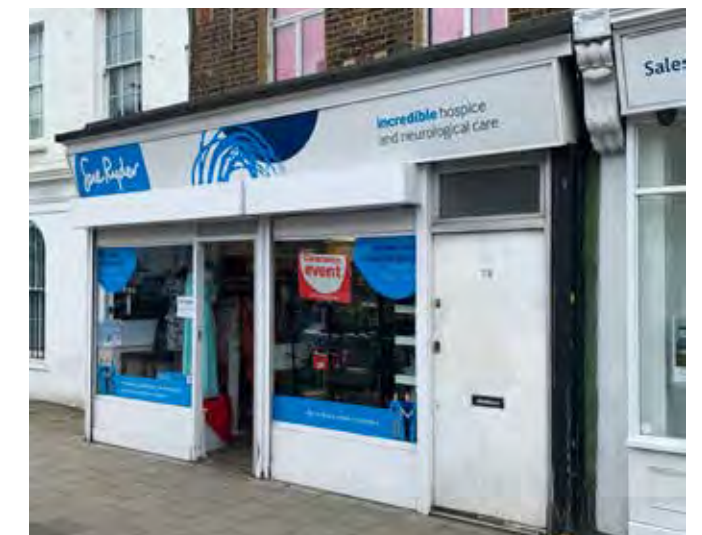
72 Essex Road, shop extension built tight on centre of party wall (or even over the line) not to inside as normal with shops. Roller shutter box extends in front of neighbours window!!
