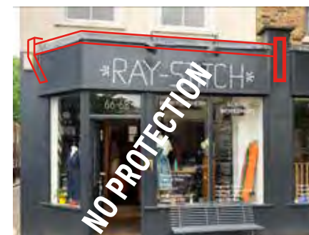
68 & 66 Essex Road, Cornice and Brackets missing
