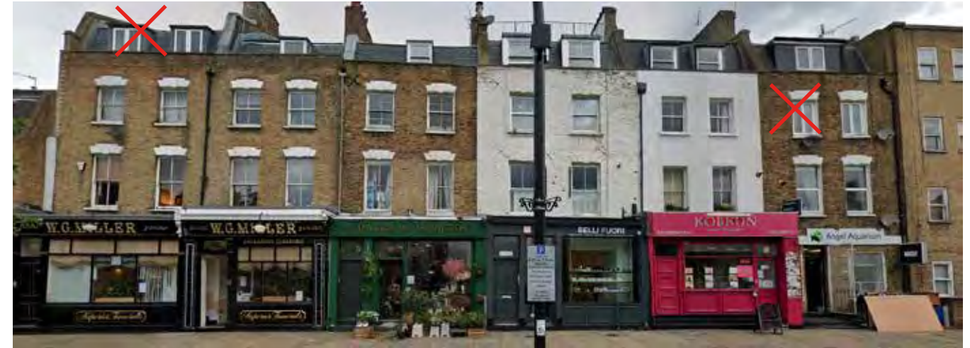
93, 95, 97, 99, 101, 103, Essex Road. Mismatched & Dormers compromised. Suit 2 over 2 triple glazed.
