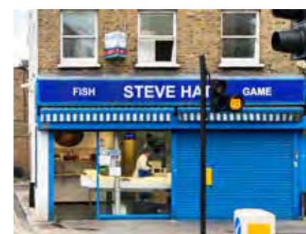
88 Essex Road, roller shutter no stall riser, brackets, cornice.
