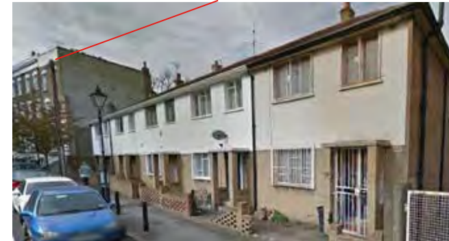
2, 3, 4, 5, 6 Dagmar Terrace /rear garages Lost heritage 4 storey terrace infill with out of scale 2 storey modern terrace damaging the Conservation Area. Poor windows and details suitable for external insulation, new windows, and additional storeys.
