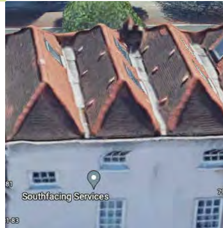
M pantiled roof. Ridge perpendicular to facade
