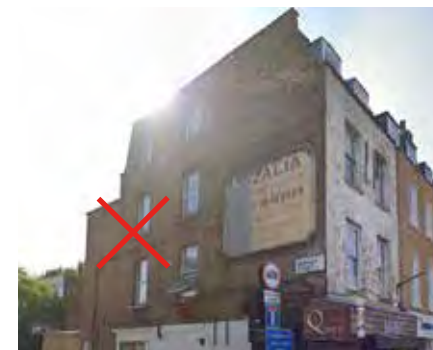
78 Essex Road, Modern rebuilt Victorian, windows compromise heritage suit 2 over 2 sash triple glazed
