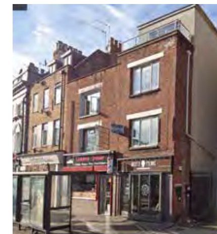
63, 65 Essex Road Poor windows and building massing at roof level suitable for external insulation and new windows
