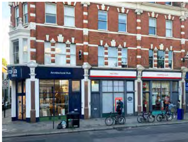
May 2022 , 159, 160, 161 Upper Street double glazed shopfronts with heritage details rebuilt
