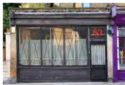
63 Cross St, House,return Shop, replace grills for a better street
